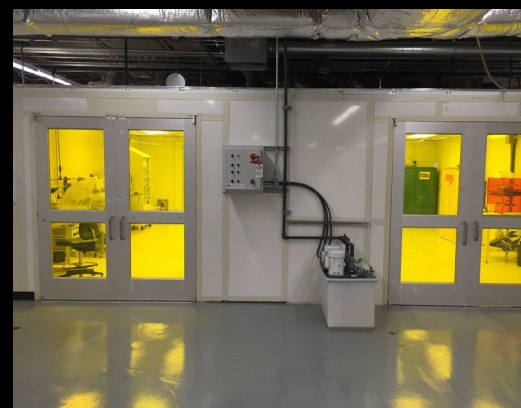
Photo Lithography Lab window coated with UV/white light eliminating film
